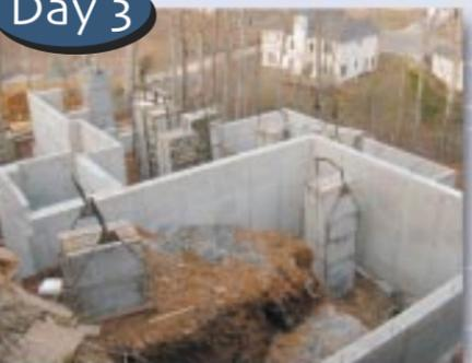
**Wednesday** – The crew returns, removes the wall forms and the project is ready for the next stage of construction. A three day timetable on the foundation walls is fairly typical. A similar wall of concrete block may have taken up to five days or more.
